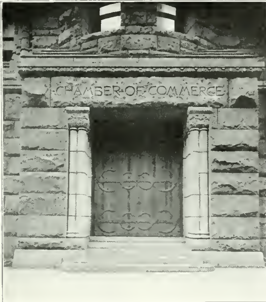
Main Entrance. To Corridors, Stairways and Elevators.
